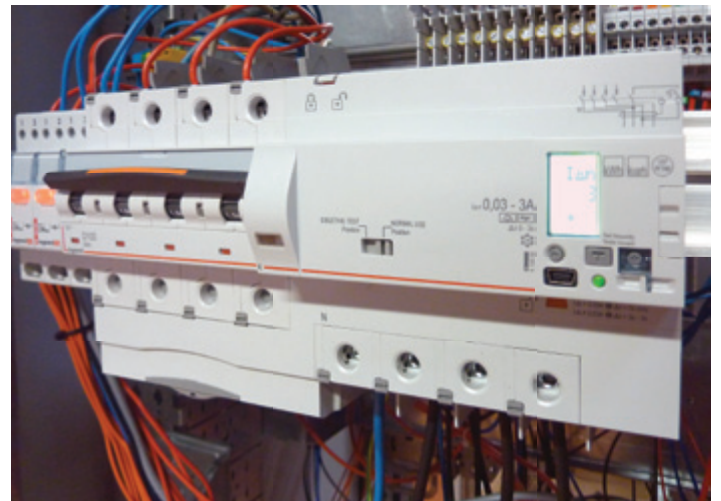
The add-on module with integrated measurement can be used with DX 3 circuit breakers with 1.5 modules per pole.
